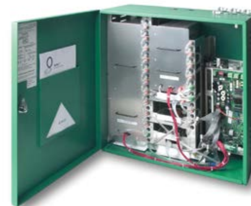
Figure 6. Aircuity Sensor Suite Used for Demand Control Ventilation (DCV)
